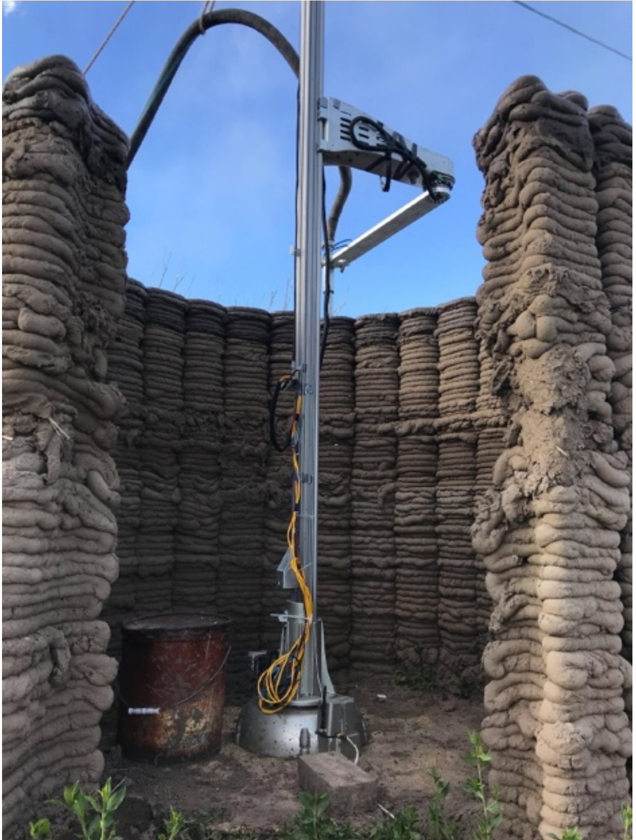
Figure 6. The construction of 3D-printed “horno” shelter structures south of the Mexico/US border
