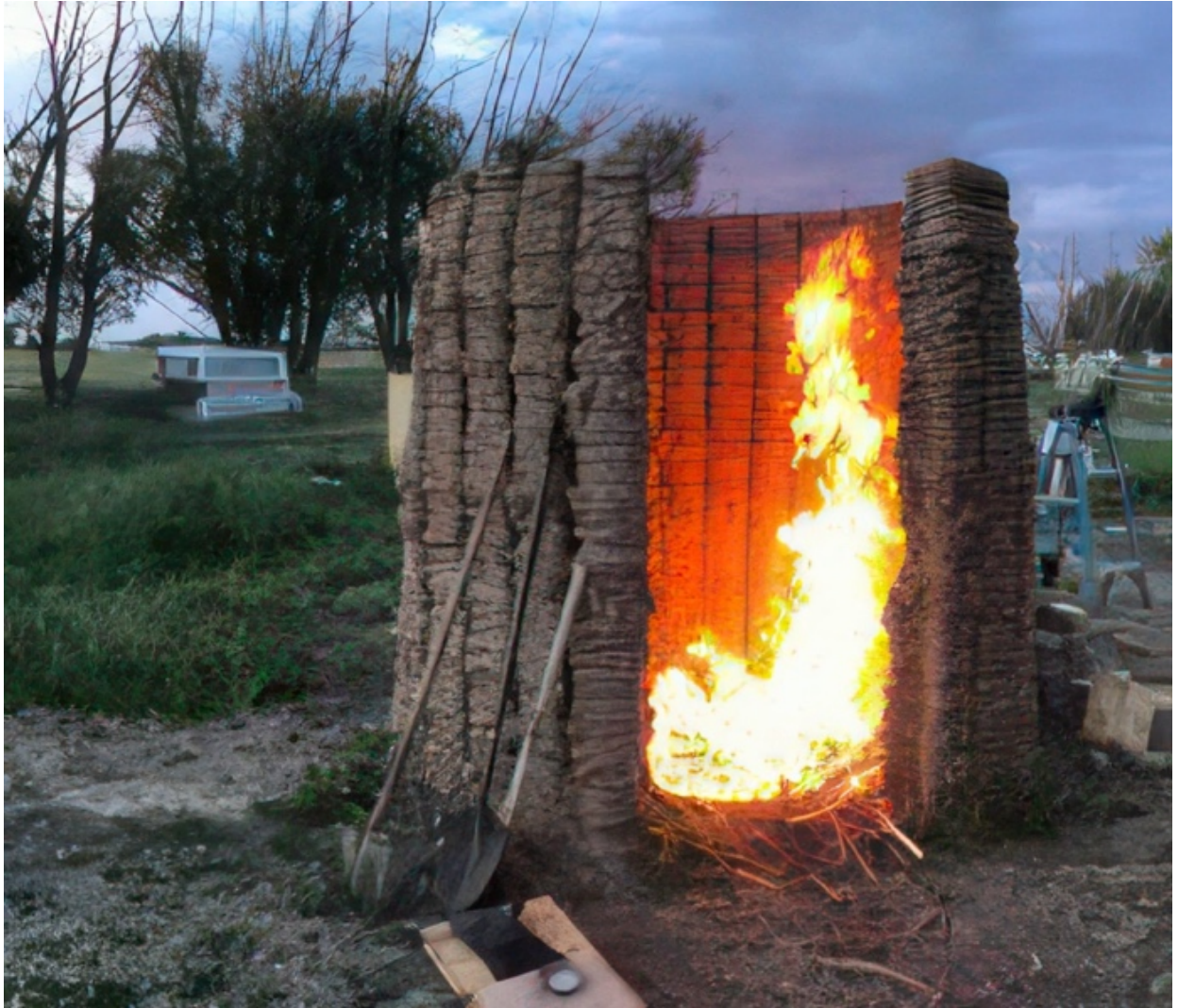
Figure 7. The construction of 3D-printed "horno" shelter structures south of the Mexico/US border
