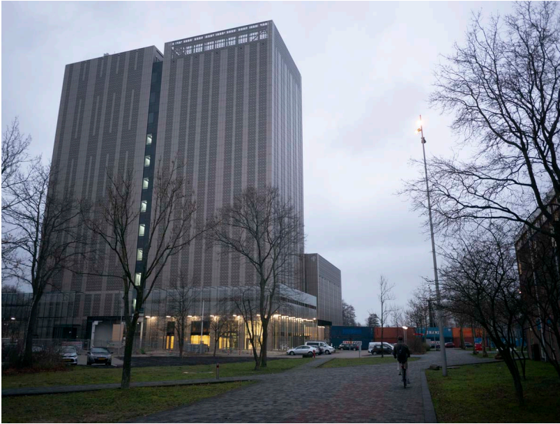
Figure 3: Amsterdam Data Tower, note the containers at lower right, photo: Benj Gerdes
